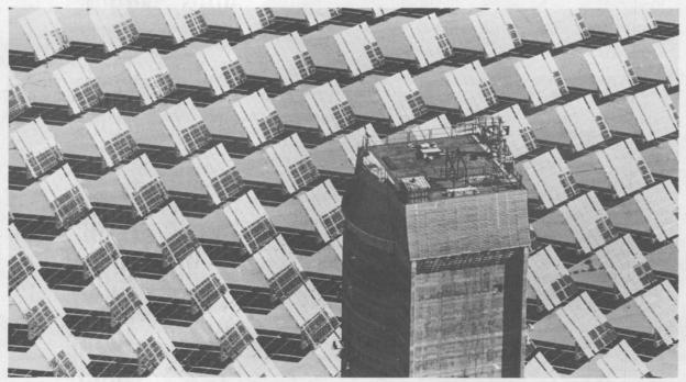
OUT STANDING IN ITS FIELD — Sandia's Solar Tower Facility stands out in a field of heliostats. The heliostats (motor-driven mirrors that adapt to the changing position of the sun) focus sunlight on the top of the tower where high-intensity-light and thermal experiments are conducted.
